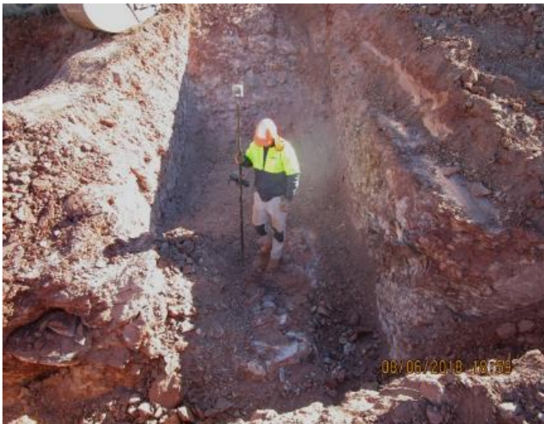
Figure 9-1. Measuring trench bulk sample.
