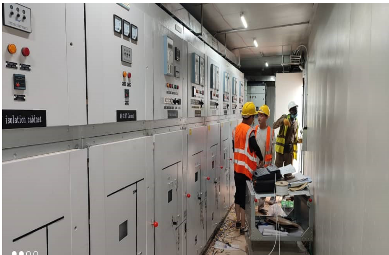
Completion of HV cabinet switch gear room
