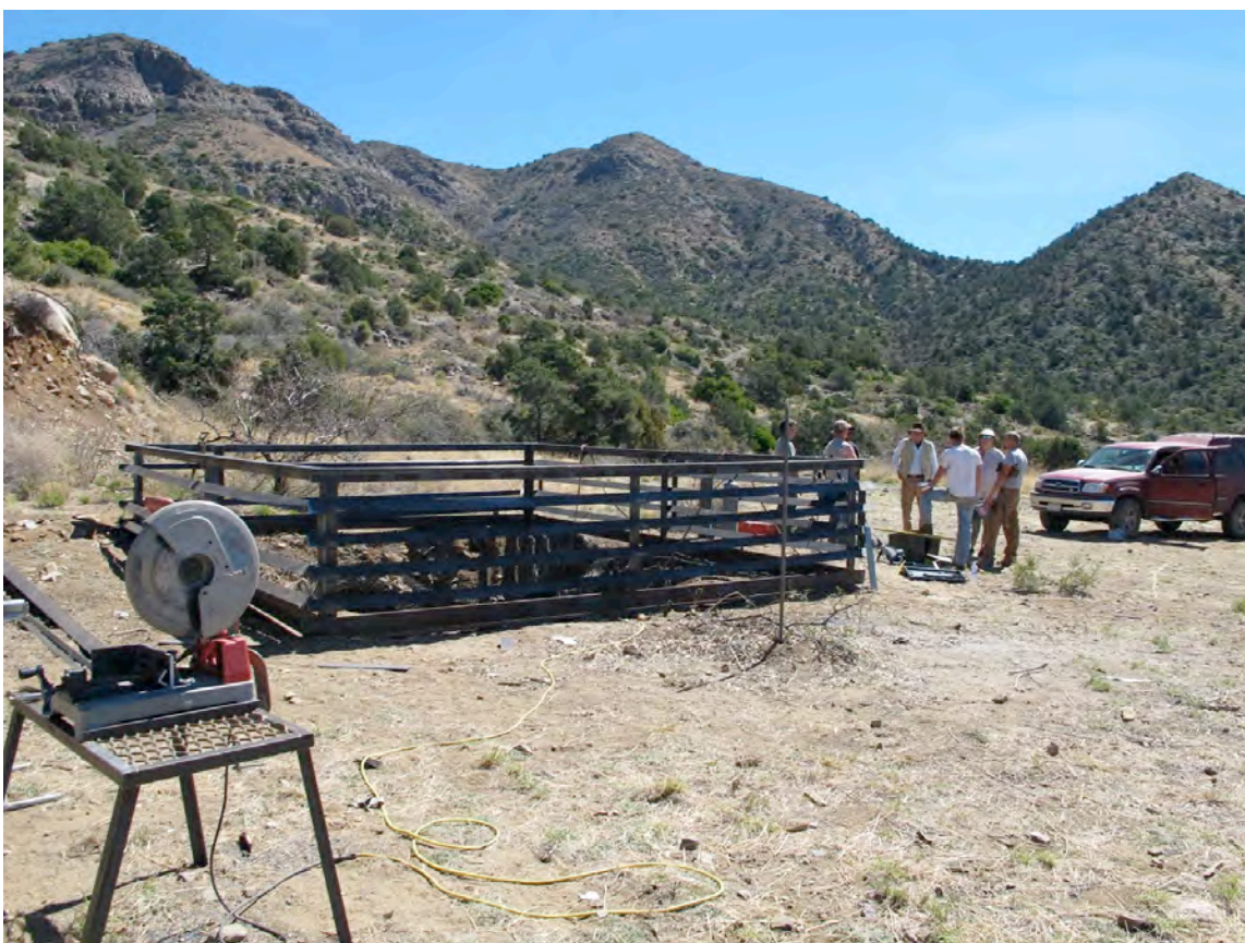
Figure 9: Rehabilitation of the McMorris shaft, Richmond Basin
