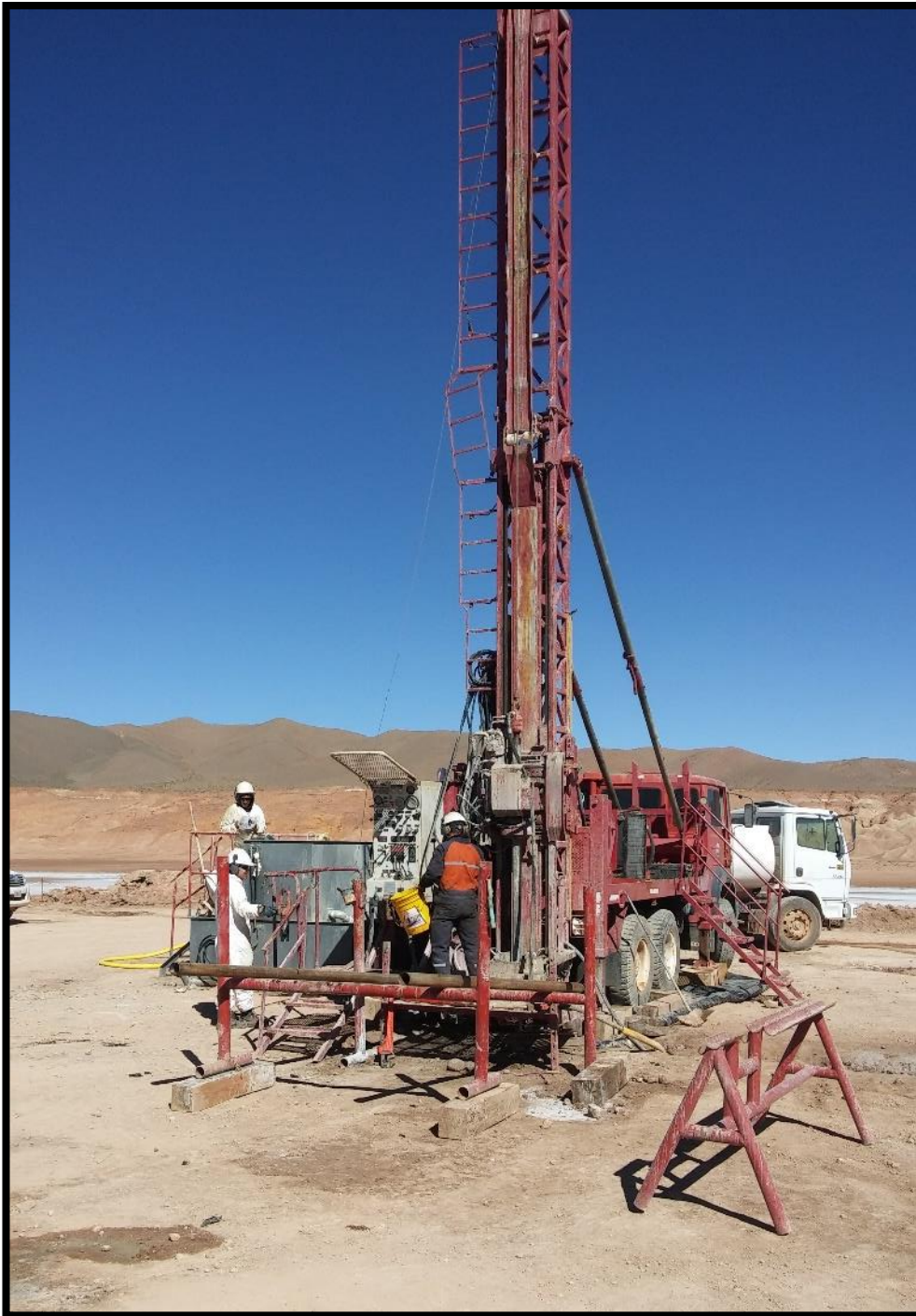
Photo 1: Drilling rig using the diamond method with tricone adaptation.
