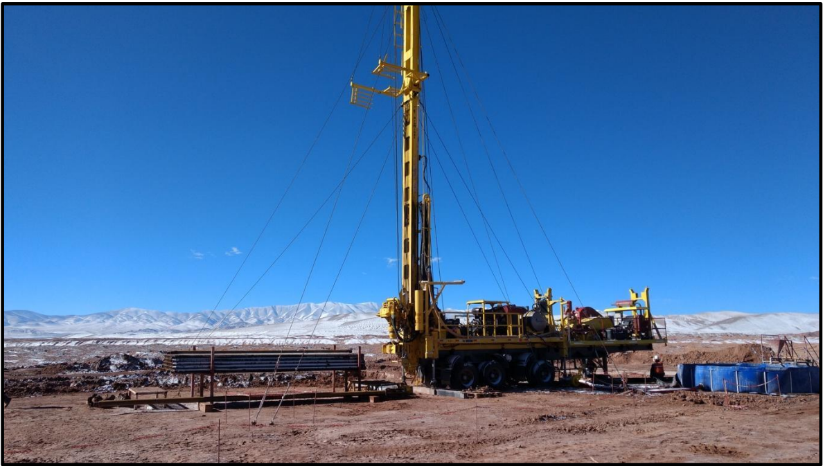
Photo 4: Platform and drilling tower for the PP-03-2019 well.
