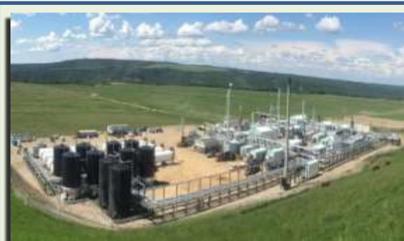
13-25 West Doe Plant
