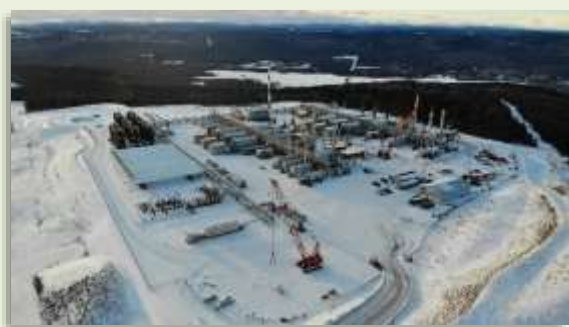
Gundy Gas Plant (Ph 1 & 2)
