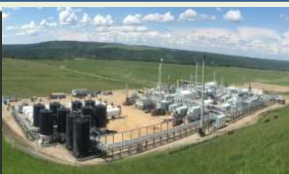
13-25 West Doe Plant
